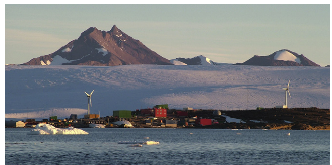
Fig. 4. Wind Turbines at Mawson Station. Photo by Peter Magill.
